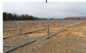
Pose des structures
