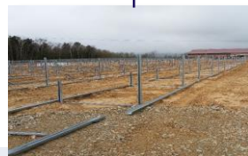
Pose des structures
